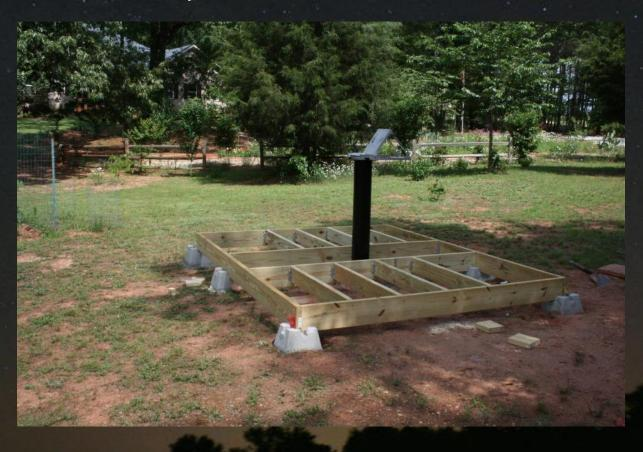
The cut out for the pier was extended so it would have additional room to put my batteries below the floor.
