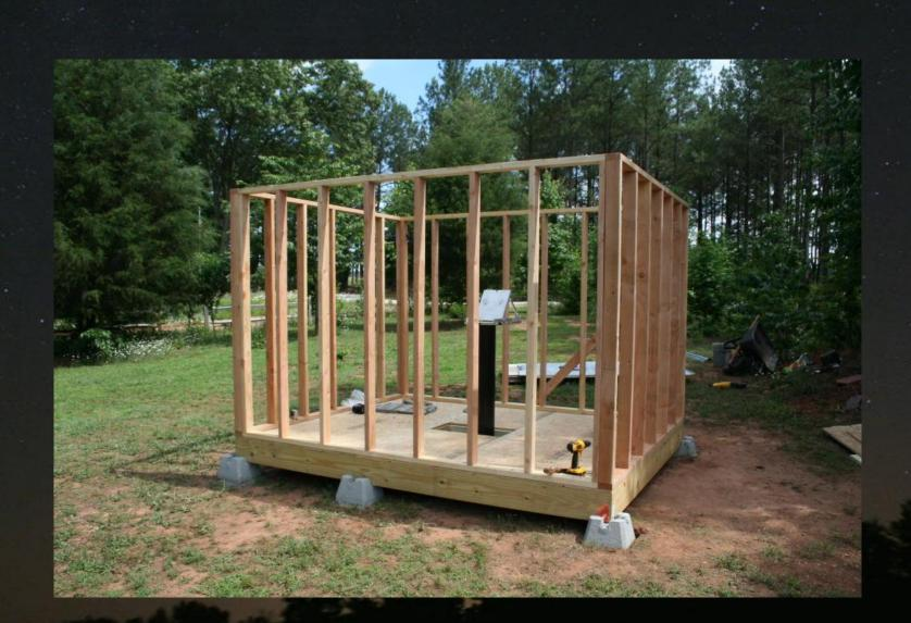
Next the wall segments were transported to the site, setup, checked for square and bolted together with two bolts on each side.
